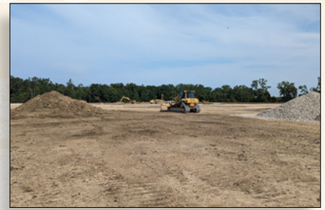
Breaking ground on the new Municipale Community Center!
